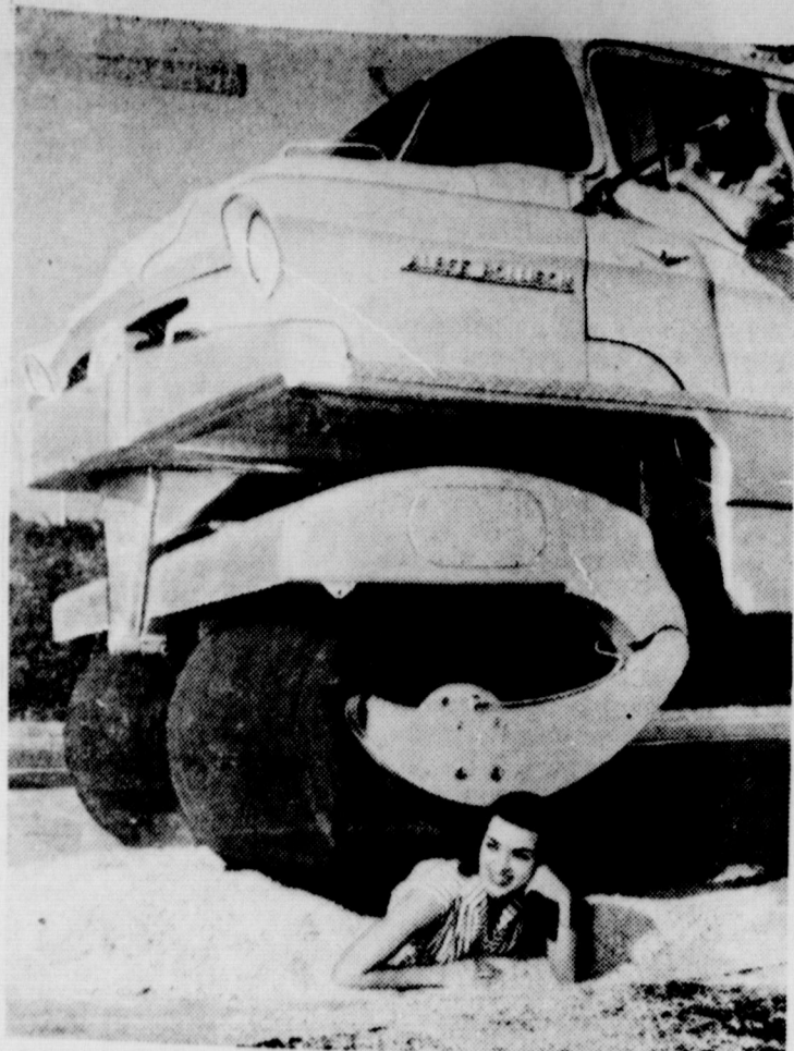
FEELING NO PAIN — Smiling Cindy O'Hara, 18, "Miss International Auto Show," bears up very well under the strain as seven tons of truck rolls over her in San Francisco. The unusual vehicle, which moves on huge, sausage-shaped pneumatic pillows instead of conventional wheels and tires, is called the Rolligen. On display at the 32nd annual San Francisco International Auto Show, the truck is able to "absorb" rocks and other obstacles (like Cindy) by "flowing around them." It is able to carry heavy loads over very rough ground.
