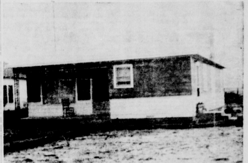
THE NEW BILL. ATHERTON HOME: This very attractive home is one of the latest additions to Canadian street. Clarence Robison was the contractor and the Wheeler Lumber supplied the materials. Bill's parents, Mr. and Mrs. Floyd Atherton are living in the new home.
