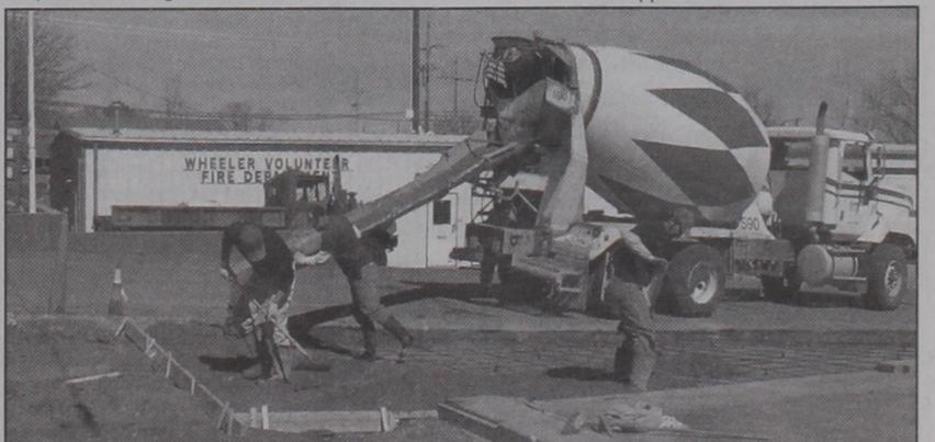
**APPROACH:** The approach to the new Wheeler Volunteer Fire Department parking garage was poured Friday afternoon. The slab for the 40’x60’ building is already in place. Erecting of the new structure should be under way, weather permitting. BMC Exteriors, Inc., of Wellington is the contractor.
