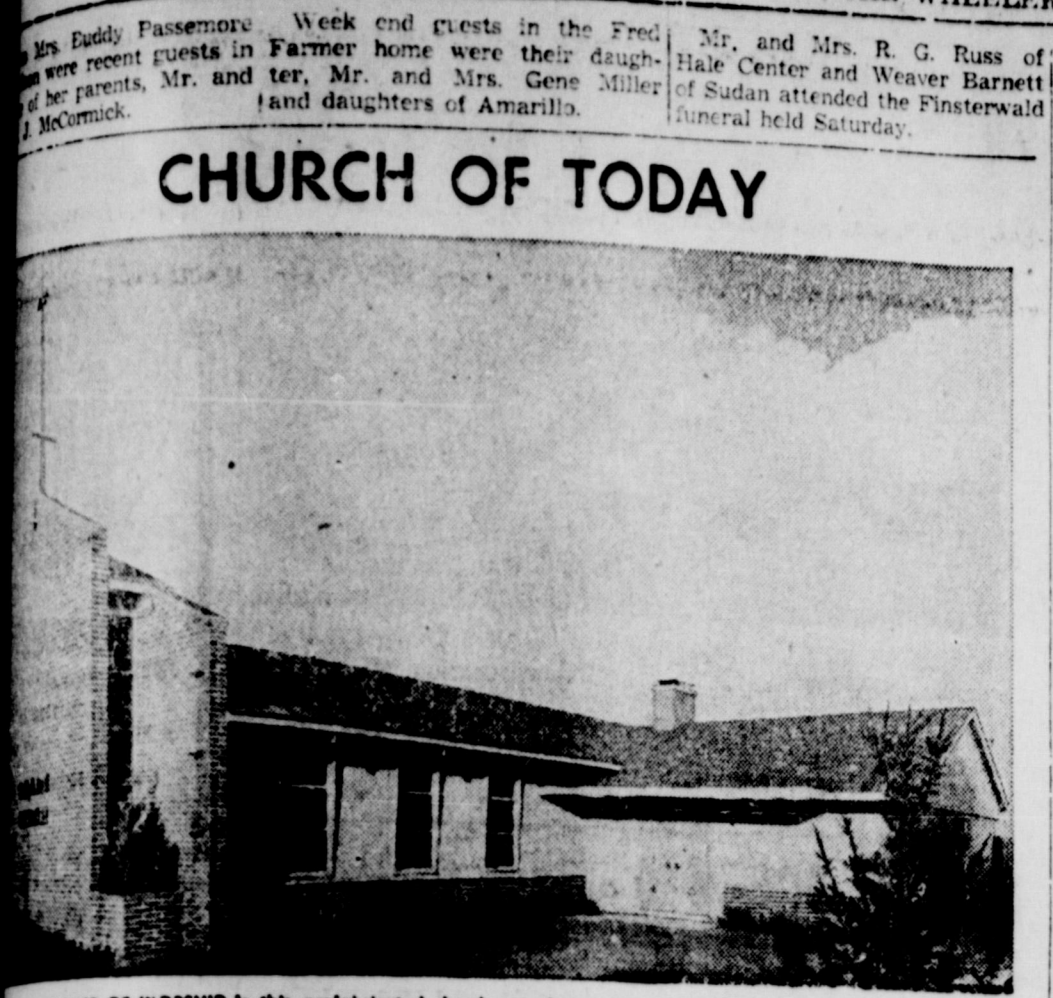
CHURCH OF TODAY is this prefabricated church manufactured by United States Steel Homes, Inc., the house of U. S. Steel corporation, at its ultra-modern plant in New Albany, Ind. Many of the churches already have been erected in various localities of the nation. Due to mass production techniques, the churches are erected speedily and without loss of strength or quality. All are expandable and, due to panelization, floor plans may be changed. The church pictured above was designed by William M. Cooley of Chicago, A. I. A.
