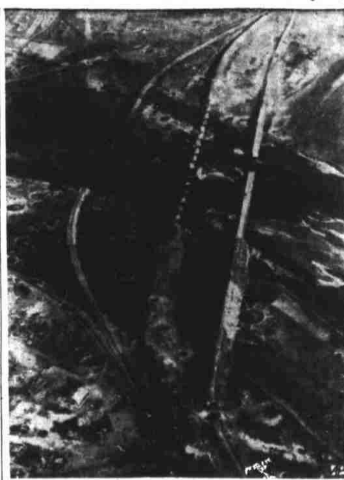
Three Down This bridge complex near Sin'p'o midway up the East coast of North Korea, has been blasted into idleness with Navy bombs of Air Group Seven from the aircraft carrier USS Bon Homme Richard. (AP Wirephoto).
