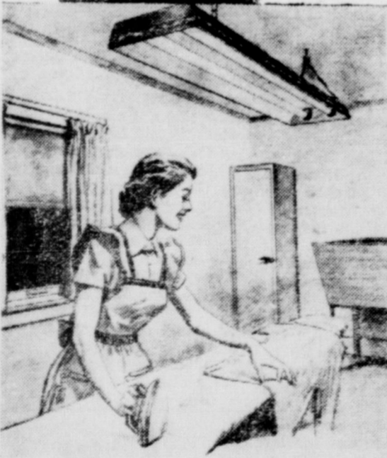
For ironing with a ceiling light you can use either of two fixtures. The one shown is a hanging fixture using two 25-watt fluorescent tubes. Or use a 150-watt silver-bowl bulb in a round metal reflector. Center fixture directly over the board.
