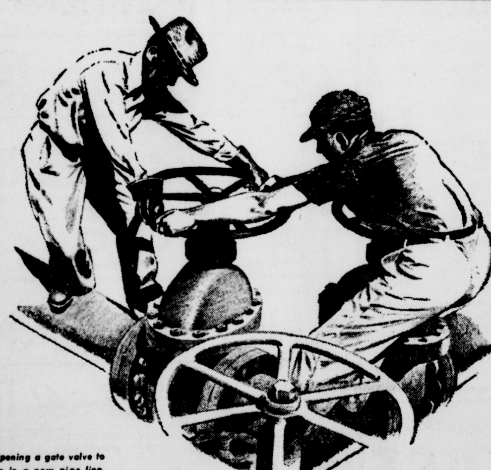
Opening a gate valve to tie in a new pipe line.
