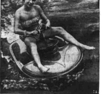
WATER SKIMMER — A German girl scoots on West Berlin lake in plastic craft propelled at top speed of 10mph. In absence of driver power shuts off automatically.
