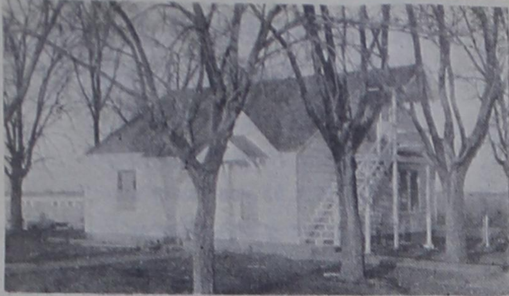
Stop by and check the remodeling in progress. Owner will help you get into this house.
