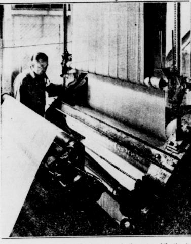
Third largest single outlet for cotton is the automobile tire industry. Shown above is a view of the National Cotton council's new tire cord going through a gum-dipping process employed in a large tire factory. The new tire cord, perfected by the Council's Cotton Research foundation as an answer to the threat of rayon in the tire industry, has a tensile strength 300% as great as that of conventional tire cords. It is being used extensively in the manufacture of heavy duty truck and bus tires.
