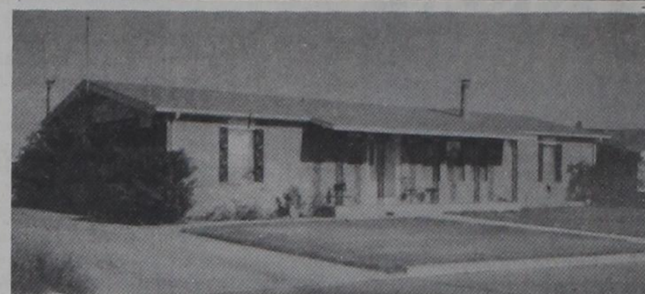
#113 Three bedroom, two bath brick home with fireplace and double garage. 1314 S. Canadian St.
