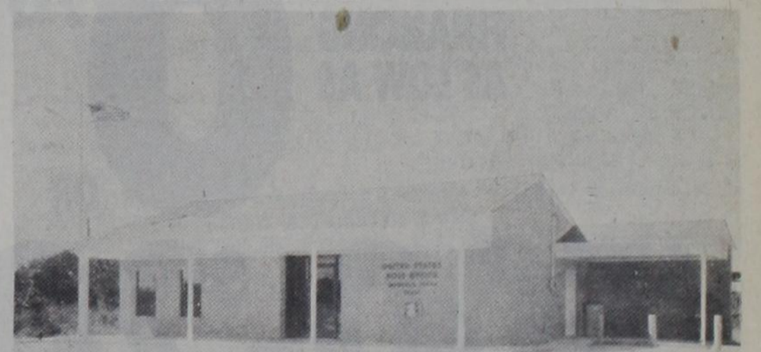
NEW BUILDING: An open house was
