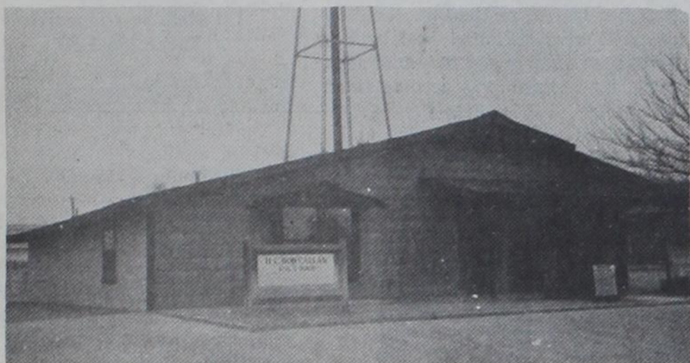
Office building—Excellent location.
