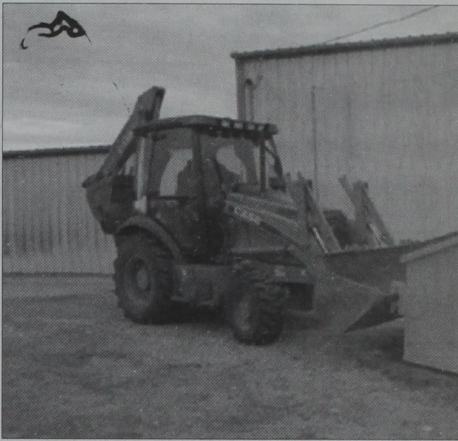
NEW DUMPSTERS: Water Superintendent Paul Arganbright is shown here setting a new dumpster. The city will take over the trash pickup beginning the first of the year. A new truck and new dumpsters were purchased. When Paul finishes, he will have set 300 dumpsters.
