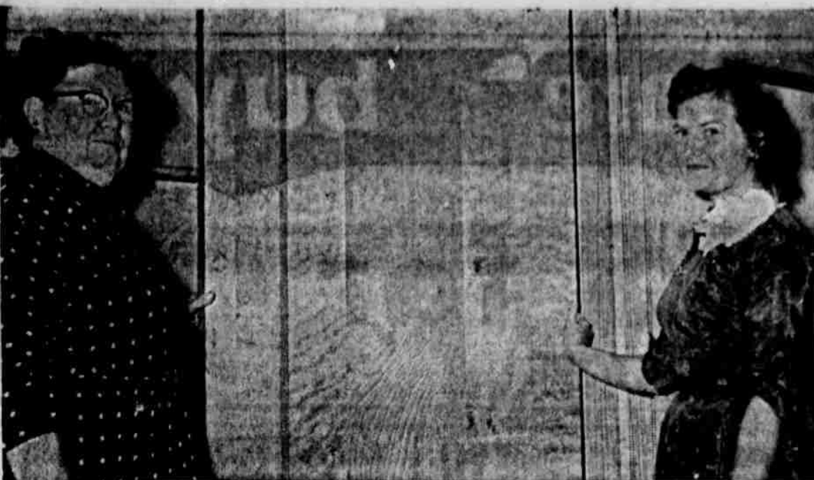
MRS. OLA JONES, left, math teacher, and Mrs. Billy Beard, home economics teacher in Sudan schools, view the sliding closet doors in the bedroom of the new home economics cottage of the Sudan schools. The cottage is in the final stages of completion with work on the interior now underway. The cottage contains a living room, bedroom, hallway, display case, bathroom, sewing room, fitting room, and kitchen units. (Scott Photo)
