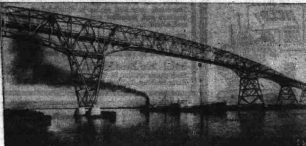
TALL TALES IN TEXAS concern above $2,750,000 span—one of the south's tallest highway bridges, to be opened to traffic in September. The toll-free bridge, crossing the Neches river at Orange and Fort Arthur, towers 230 feet above the water, at its highest point. The main span provides a clearance of 176 feet above water. Structure is 1 1/4 miles long.
