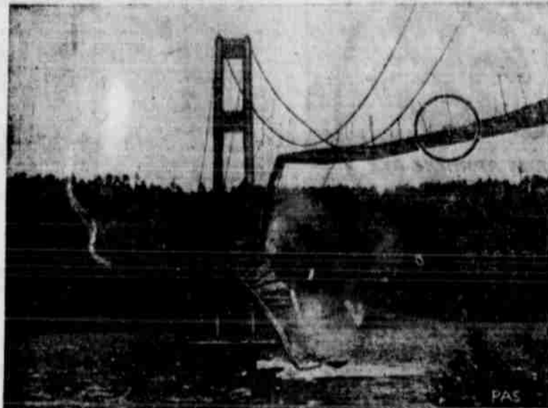
TACOMA, Wash. . . . Like a strip of cloth ripping in the breeze, the center span of the Tacoma Narrows $6,500,000 bridge writhed and twisted under the force of a forty mile wind and collapsed into the channel below. This remarkable photograph was taken just as the bridge collapsed. Built with P.W.A. funds, an investigation into the causes of the collapse is now being made. Circle shows an automobile on the bridge. The driver crawled back to safety.
