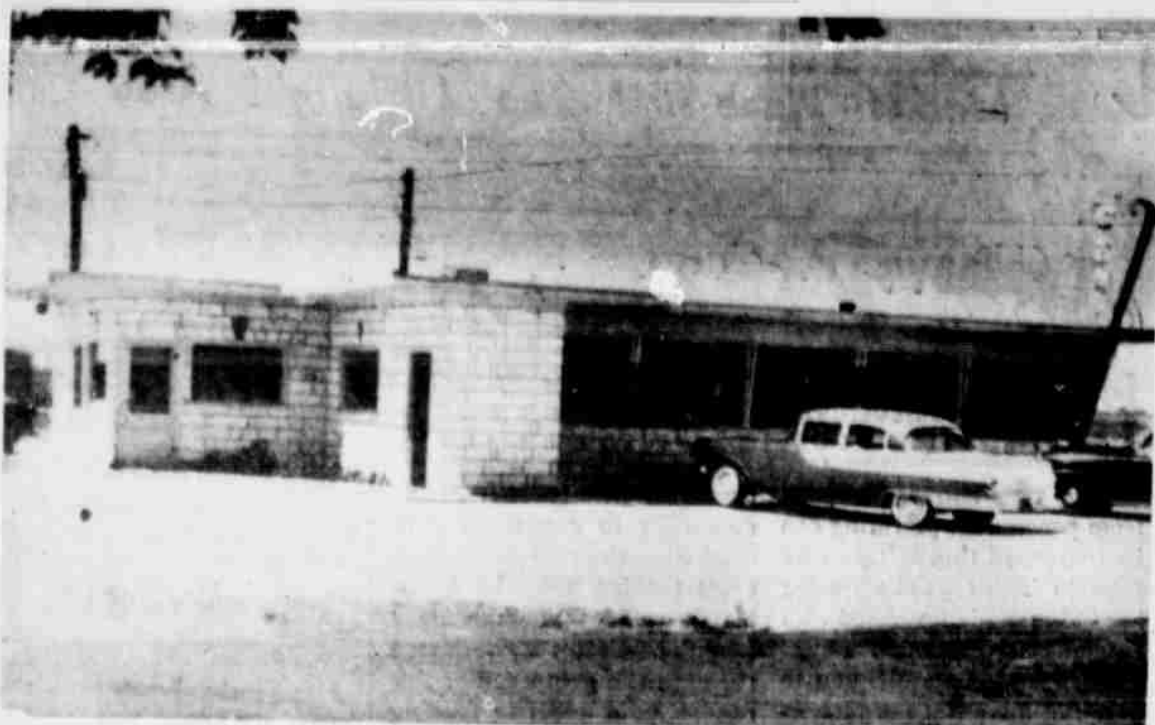
THE MODERNISTIC new building which houses Clay's is finished with natural stone. It is located one mile east of Littlefield on the Lubbock Highway.
