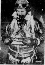
George H. Dorsey, test pilot for a large airplane manufacturer at Dayton, Ohio, is shown wearing high-altitude equipment, including the new harness designed for carrying the emergency oxygen supply on the chest. This permits free movement within the close quarters of a single-seater pursuit plane.
