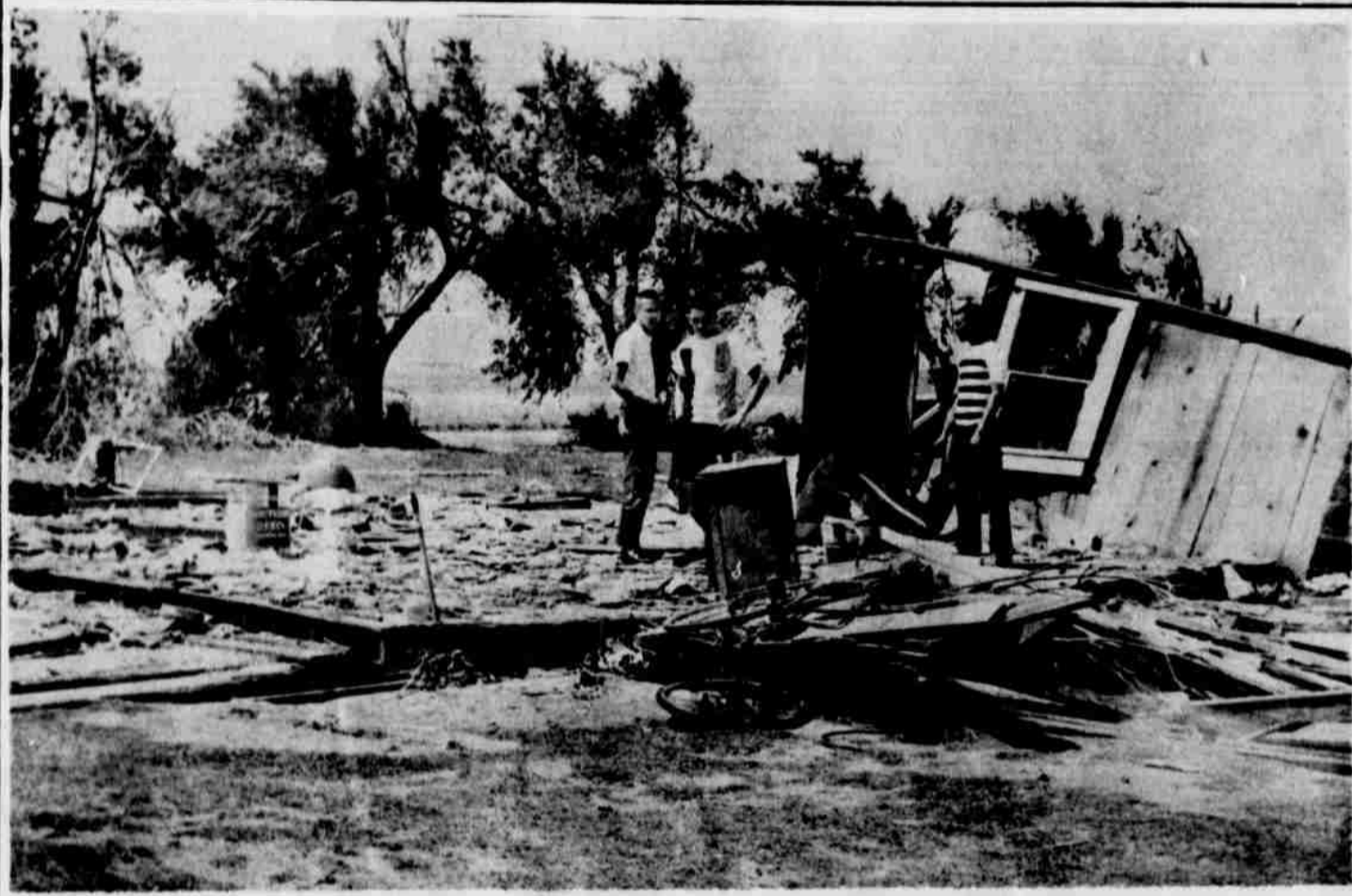
HOME IS DESTROYED BY TORNADO--Above is all that remains of the Allen Roberson home located four miles north of Sudan after Saturday's tornado swept through it. Roberson and his family had just taken his family to shelter when the storm struck. Other storm damage pictures can be found inside today's issue.
