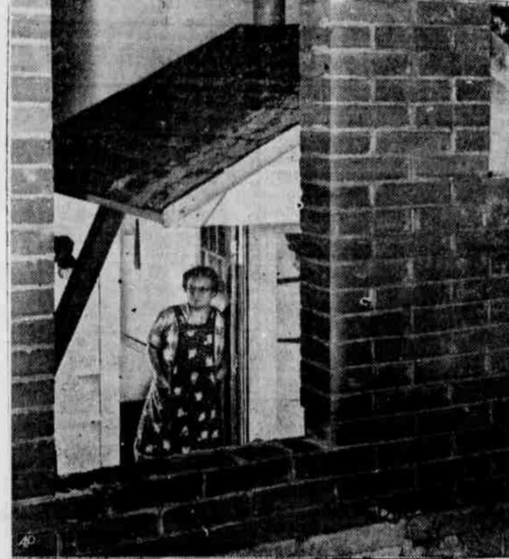
OLD HOUSE inside the growing new structure.
