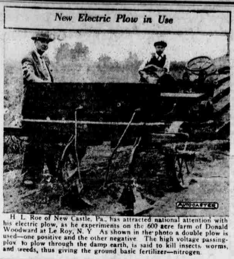
New Electric Plow in Use H. L. Roe of New Castle, Pa., has attracted national attention with his electric plow, as he experiments on the 600 acre farm of Donald Woodward at Le Roy, N. Y. As shown in the photo a double plow is used—one positive and the other negative. The high voltage passing-plow to plow through the damp earth, is said to kill insects, worms, and weeds, thus giving the ground basic fertilizer—nitrogen.
