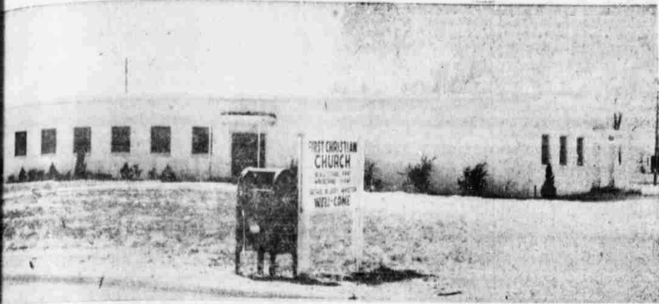
FIRST CHRISTIAN CHURCH in Littlefield is located on Phelps Avenue, and was completed late last year. It is modern in design and contains a sanctuary, classrooms and a banquet room for large gatherings. (Staff Photo)
