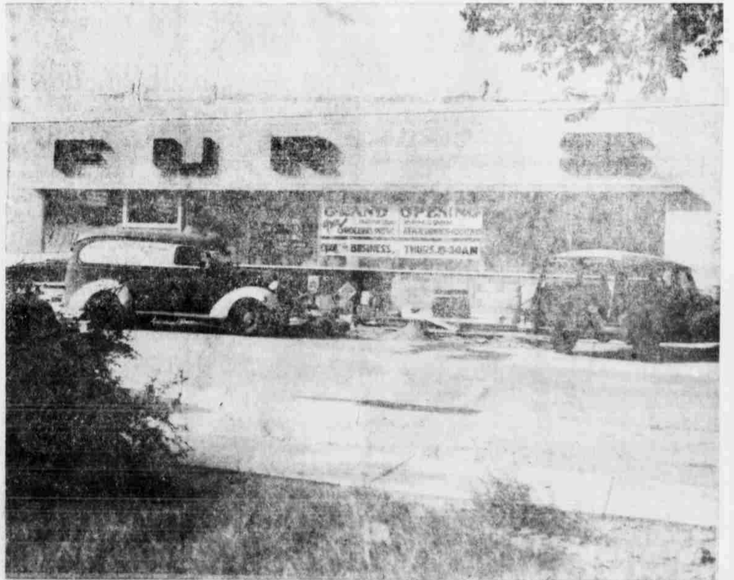
Here is the "New" Furr Food Store under construction in 1949
