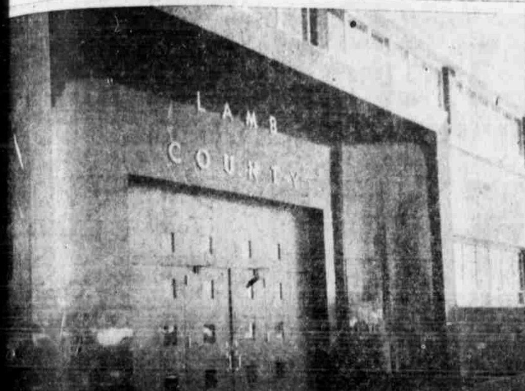
ENTRANCE OF THE NEW LAMB COUNTY COURTHOUSE, is constructed of dark marble, framed in dark red brick, with light stone trim. Aluminum doors and the name add a touch of brightness to the modern entrance. (Staff Photo)
