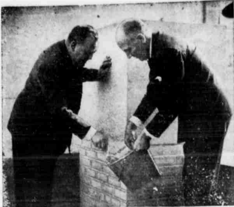
CORNERSTONE OF U.N. permanent headquarters is cemented into place by U.N. Secretary-General Trygve Lie, wielding trowel at ceremony on United Nations Day, 24 October 1949. Ready with mortar is architect Wallace K. Harrison, who directed planning.
