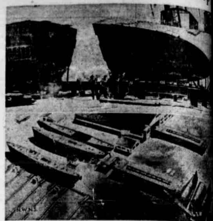
Above you see one phase in the assembly of U. S. submarines built by the Dravo corporation of Pittsburgh, Pa. The 1700-tonners are built upside down, sections being welded in that position. The sections are then braced and turned right side up. The bow and stern above is being turned over, preparatory to being joined to the station at left. Below: A wash drawing showing sub-chamber assembly just to the left of the indoor barge assembly shop at the Dravo yard.
