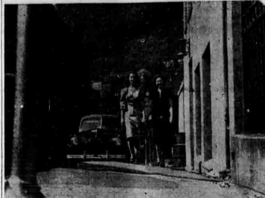
EARTH SHIFTING THREATENS TOWN . . . Two hardy members of the opposite sex, residents of Welch, W. Va., brave a stroll on the buckled streets of the town after sections of the little city started to sag alarmingly because of a mysterious shifting of the earth. Huge cracks appeared in several large buildings, and inhabitants were fearful that their homes would be destroyed.
