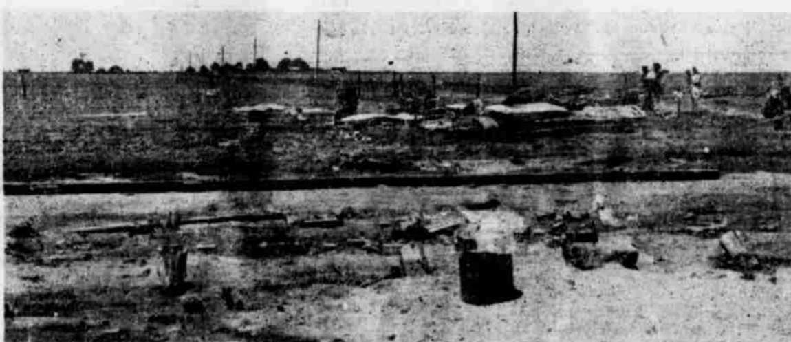
The above picture shows what is left of the A. W. Baxter home, three miles north and a mile east of Spade, on the A. P. Hutchins farm, after a tornado struck about
