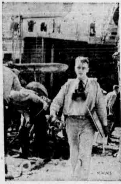
Senior pilot of a U. S. warship returns to his vessel to report to his captain on progress of the blasting of Jap bases in the Gilbert and Marshall Islands. Behind the pilot men are working to repair the damage done by a Jap bomb which hit the ship during raid which sent 16 Jap ships to the bottom.
