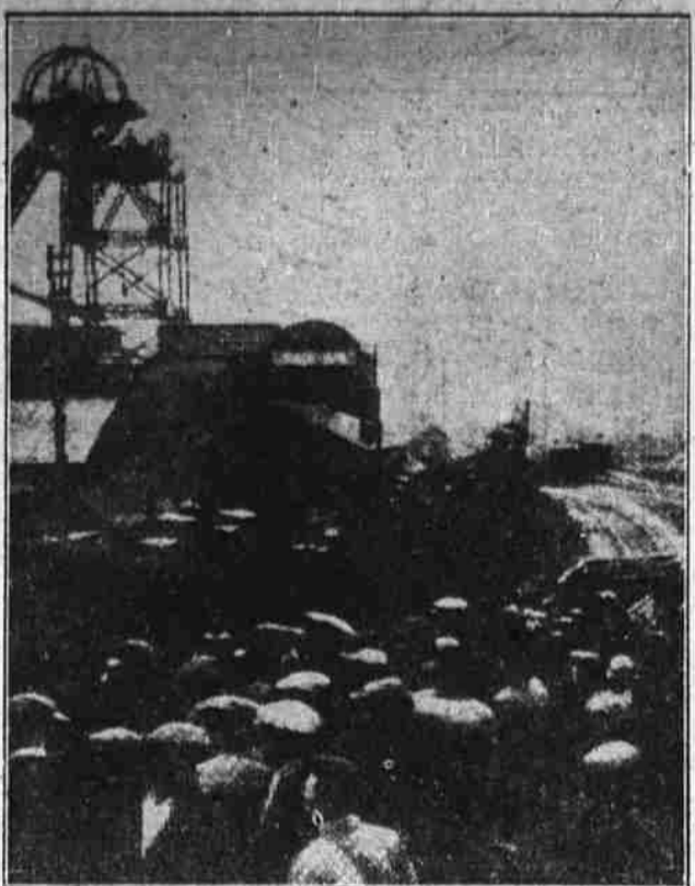
This Associated Press picture sent by radio from London shows the mouth of the Gresford coal mine at Wrexham, Wales, where it was feared upwards of 200 miners lost their lives when an explosion and fire cut off their escape. Nine hundred others in the mine fled to safety.
