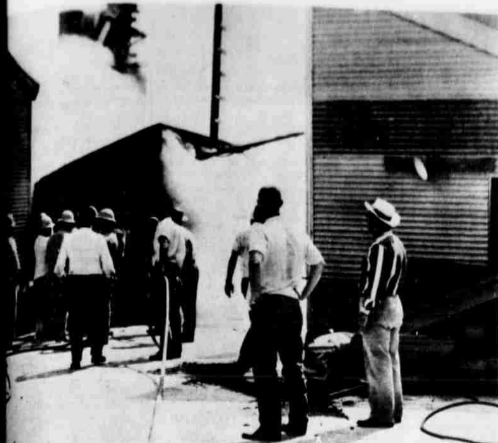
IN THE CONTROL ROOM -- A fire at the Nipak Fertilizer plant Tuesday morning caused in more than $2,500 damage to the switches and control boxes in the
