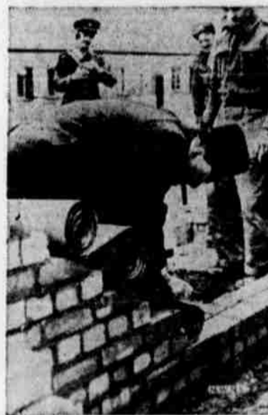
Winston Churchill at his favorite pastime—next to prime ministering—laying bricks. During a visit to an anti-aircraft battery, Churchill saw some soldiers busy building a brick wall. He took a hand. Premier Churchill holds a bricklayer's union card.
