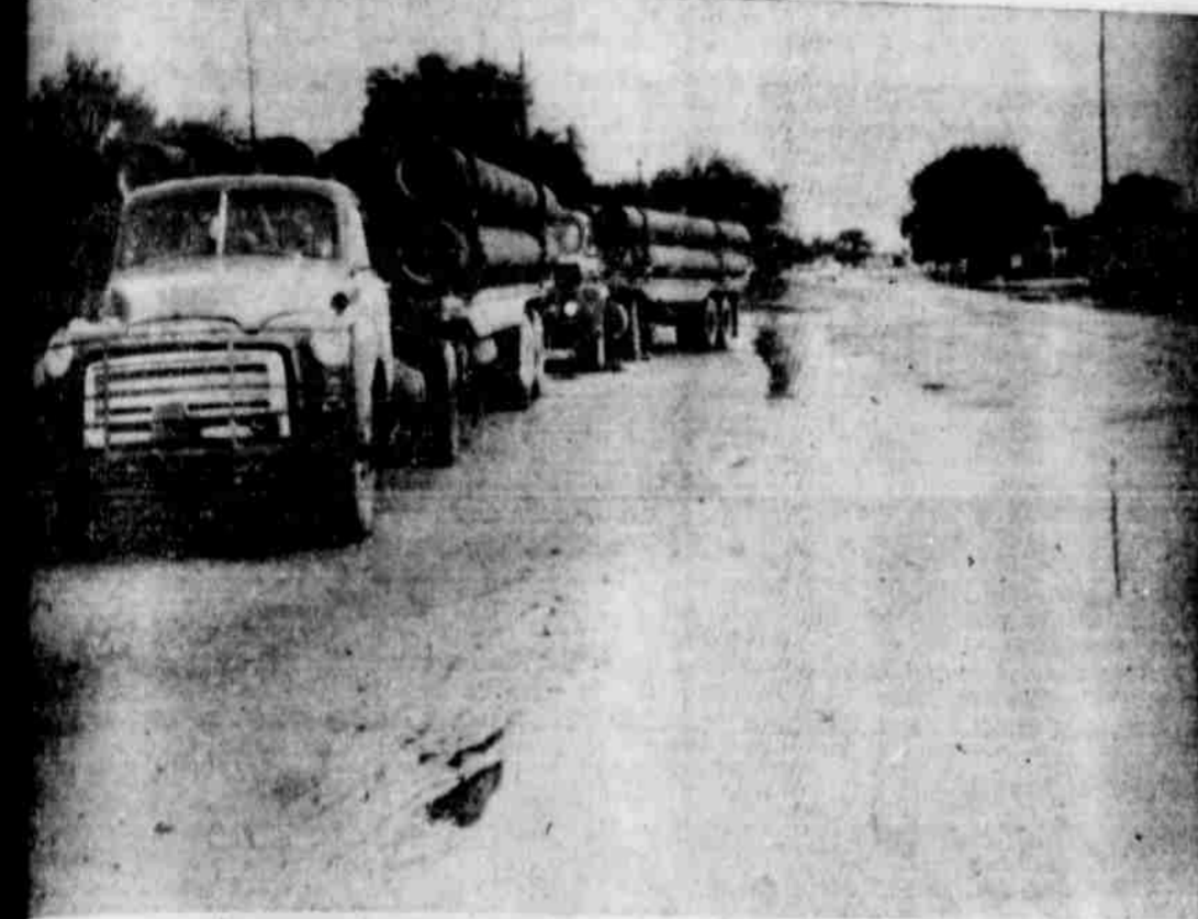
WATERWORKS PIPELINE ARRIVES DURING DOWNPOUR. The first two loads of 10 truck-loads of concrete coated steel pipe arrived in Littlefield Sunday afternoon during a downpour of rain. The pipe is for the waterworks extension from water wells 7 and 8 on the Sorrenson property, and was delivered by Gifford-Hill American Pipe Company. Workers will begin laying the pipe as soon as weather conditions permit. (Staff Photo)
