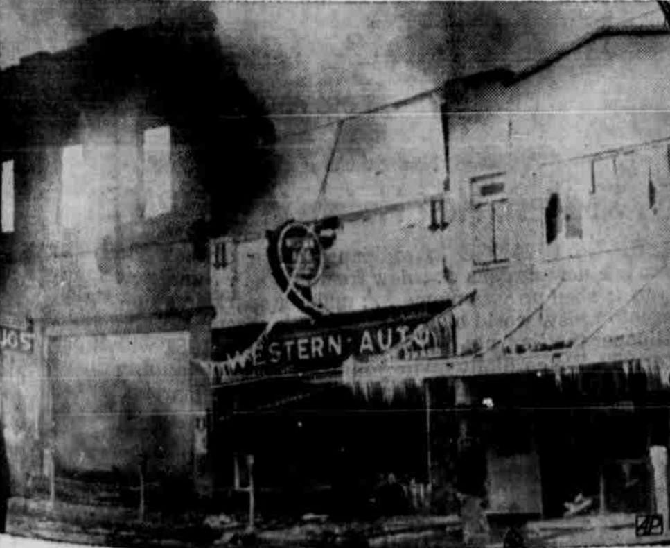
DOWNTOWN CHILDRESS — Buildings stand on downtown street after flames swept causing an estimated $1,000,000 damage. In addition to the First State Bank building, Prather-Williams Drug Store, Western Auto Store and Gem Theater (left to right), the fire also destroyed a news stand and fashion shop in the same block but around the corner. Firemen from eight Texas panhandle cities fought the stubborn pre-dawn blaze in five above zero weather. (AP) Photo
