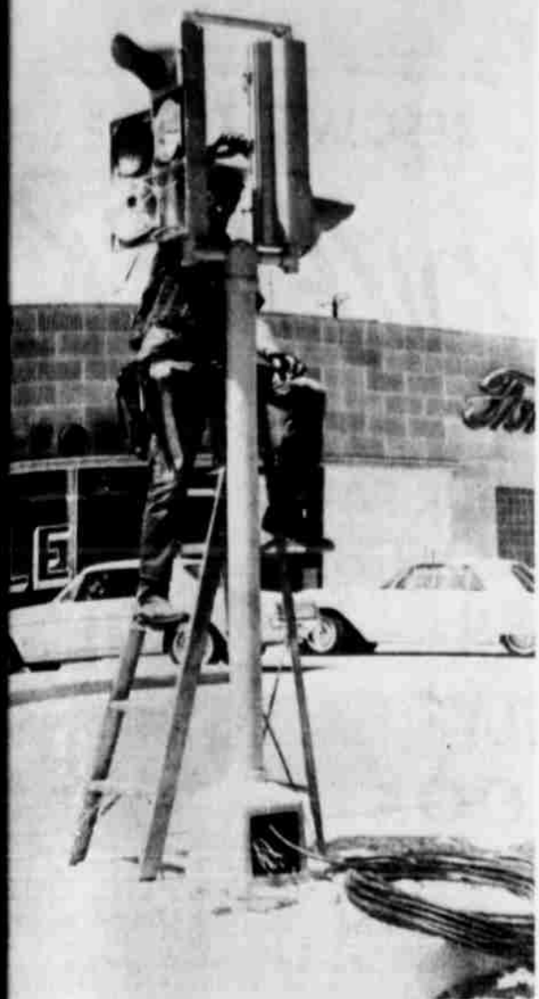
SIGNAL LIGHTS -- The new signal lights being installed on Phillips Ave. will eliminate another overhead wire across the street. An added improvement with the new lights that the green lights will be on the bottom in both directions of traffic. The first lights were installed Tuesday at Phillips and put into use Wednesday morning.
