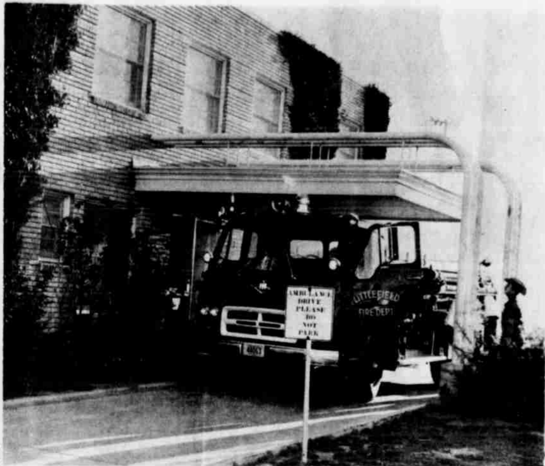
EMERGENCY ROOM FIRE -- A fire broke out in the emergency room of the Medical Arts Hospital Monday evening when a hot iron was left on an operating table. The fire, while confined to the emergency room, caused consid-
