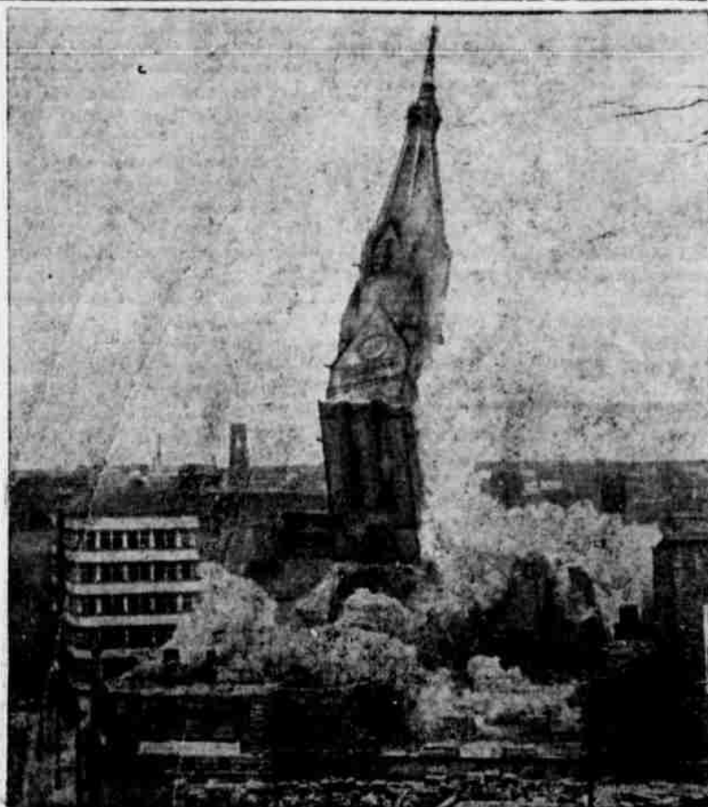
BERLIN COMMUNISTS BLOW UP CHURCH... The historic Georgian church, one of Berlin's most famous landmarks on the Alexander Platz, survived the fire and explosion of World War II. The Communists, contrary to reports by engineers, termed it unsafe and destroyed it by dynamite. Protestant leaders protested, but the demolition squad destroyed it as Communist police and Russian soldiers cowed an indignant crowd of Berliners. The church was damaged by World War II bombs.
