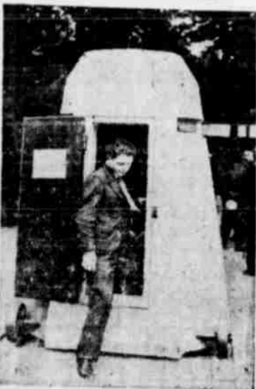
PARIS... A Parisian steps out of one of the special mobile air raid shelters made of steel, after taking shelter during an air raid.
