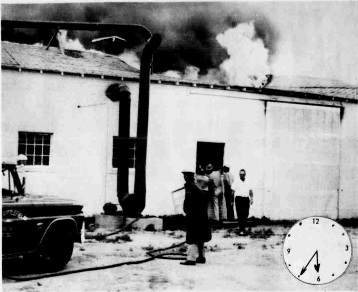
6:35 A.M. . . . FIREMEN ARRIVE AT BLAZE, AS FLAMES BREAK THROUGH ROOF OF PLANT
