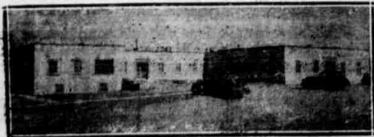
THE NEW LITTLEFIELD HOSPITAL
