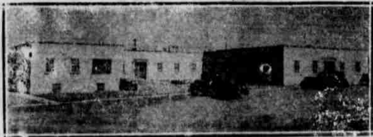
THE NEW LITTLEFIELD HOSPITAL
