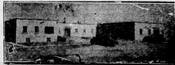
THE NEW LITTLEFIELD HOSPITAL
