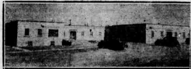
THE NEW LITTLEFIELD HOSPITAL
