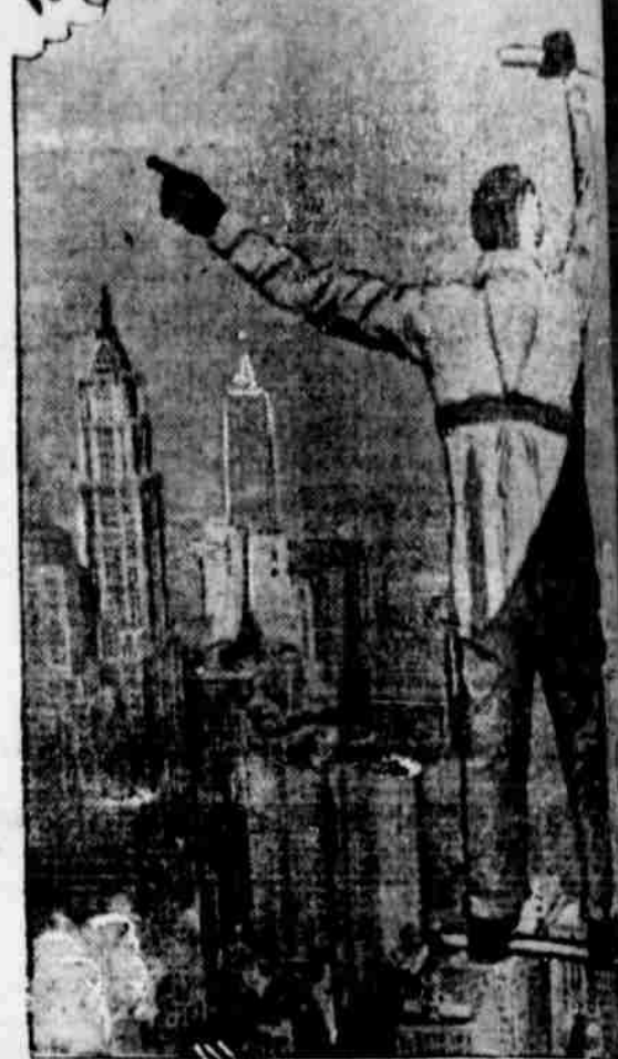
M. P. Doherty, a Brooklyn steel erector, swinging out from the new Bank of Manhattan building in Wall Street, the Woolworth Tower and the money center of the world. Stock Exchange is the low building in the center of the picture.
