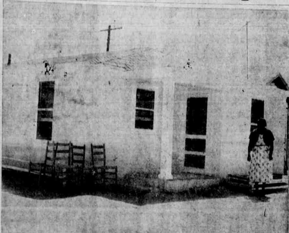
Shown above is the newly erected St. John's Baptist Church parsonage for the new minister, Rev. V. Ottis and his wife, who recently moved here from Oklahoma. The dedication service for the five room home was held recently in the St. John's Baptist Church with Rev. Walter Griffin of the Mount Pleasant Baptist Church in Lorenzo, Texas, bringing the message. Joel Thompson, secretary of the city, also made a speech to the approximately 175 people attending.
