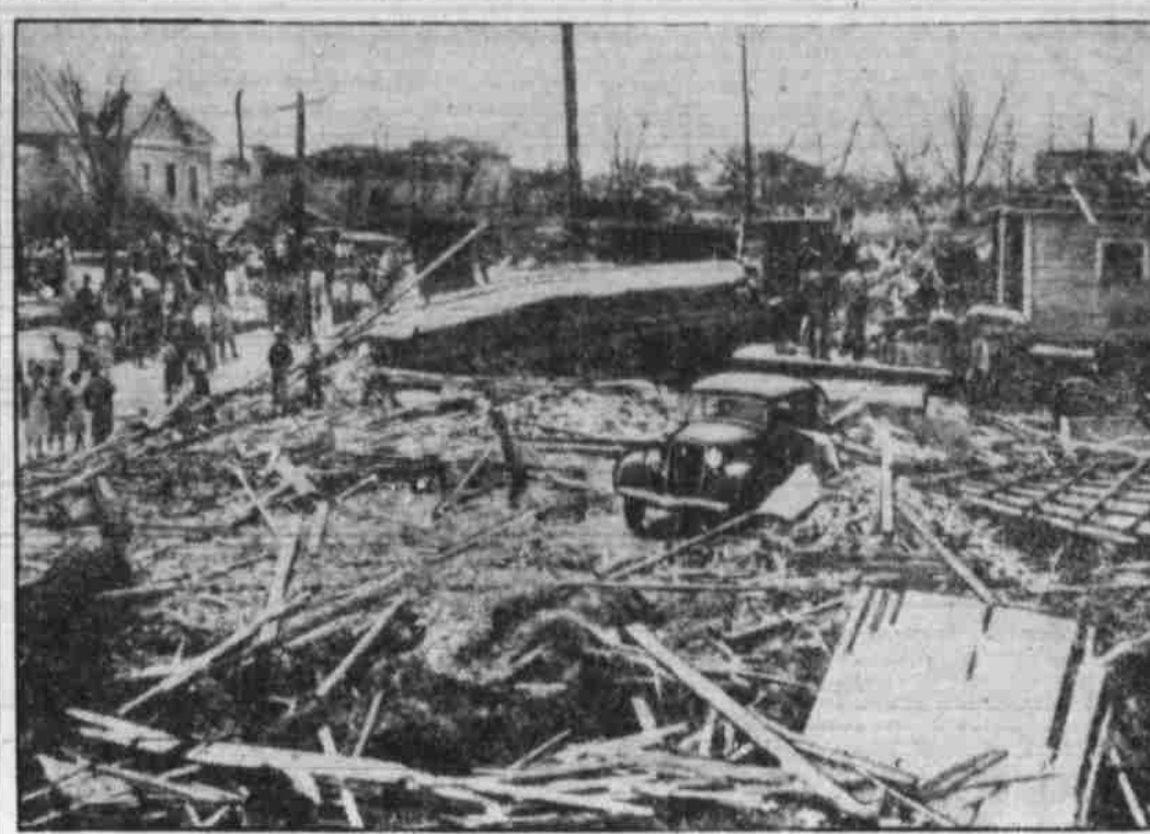
Scenes like the above were common in Georgia, Mississippi and other tornado-swept states, after a ravaging storm had taken a toll of over 300 lives and $25,000,000 in damage. The above photo is a general view of Cordele, Ga., where 19 persons were killed last week, leaving a scene of heaped debris and widespread suffering. (Associated Press Photo)
