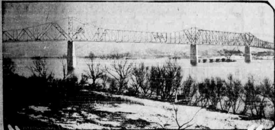
The new Madison-Milton bridge, costing $1,800,000, which shortens the distance between Indianapolis and Frankfort, the capital cities of Indiana and Kentucky, by forty miles. It also opens a new short route from Chicago and the Northwest to Florida and the South coast. The bridge spans the Ohio river between Madison, Ind., and Milton, Ky.
