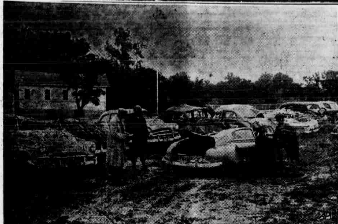
Monday's tornado at Waco, Texas, after it was pulled to a vacant lot May 11. The autos dragged from the wreckage left by the tornado are pulled to the lot where their numbers are checked for the owners who are then notified of their location. (AP Photo)
