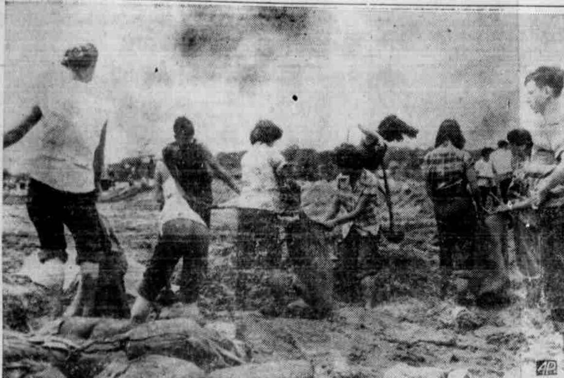
SCHOOL CHILDREN HELP —High school girls and boys, out of school because of the flood threat at Orange, Texas, help fill sandbags for strengthening weakened levees on the rampaging Sabine River. The river's crest was expected to threaten the town with severe damage. (AP Photo)
