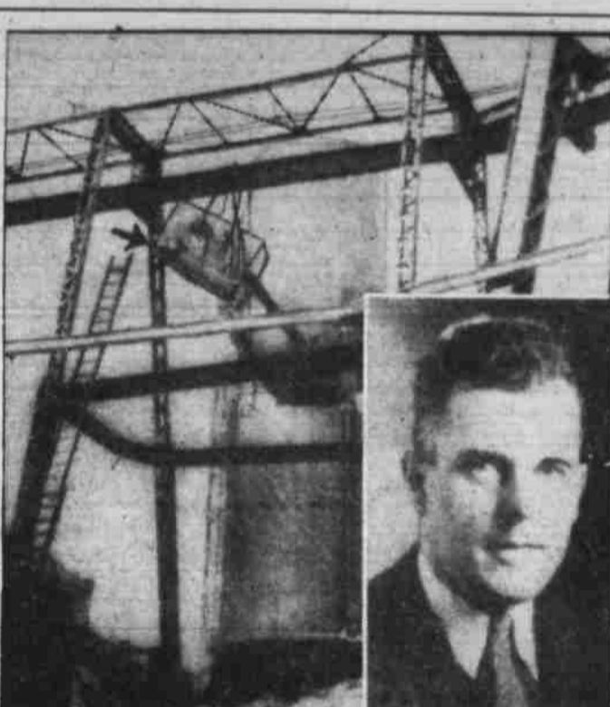
After climbing 50 feet to the top of the ladder shown above, Dr. N. Gillmor Long (insert), amputated the arm of John McCoy with a hacksaw. McCoy had been pinned to the steel girder indicated by an arrow, when the cable cab broke loose. He was improving in a Lowell, Mass., hospital. (Associated Press Photo)
