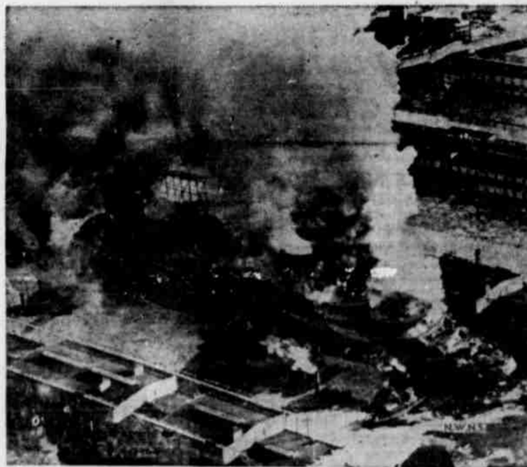
An aerial view of the $60,000,000 French superliner, Normandie, recently re-named the U. S. S. Lafayette, is shown as smoke poured out from its interior at her berth in New York harbor. Fire boats poured tons of water into the burning vessel, which finally capsized. There were 300 sailors, 400 coast guardsmen and 800 workmen aboard when the fire broke out. The navy took over the Normandie last December 16 for conversion into a naval auxiliary.
