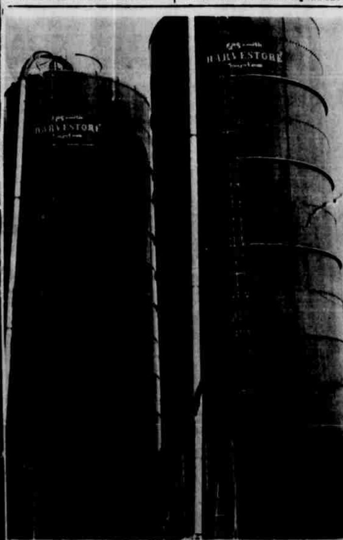
LOTS OF FEED, from 275 to 300 tons of "haylage" for cattle feeding goes into each of these two giant airtight tanks. It comes out on automatic order and is maintained in the tank at a critical 30 percent moisture content.
