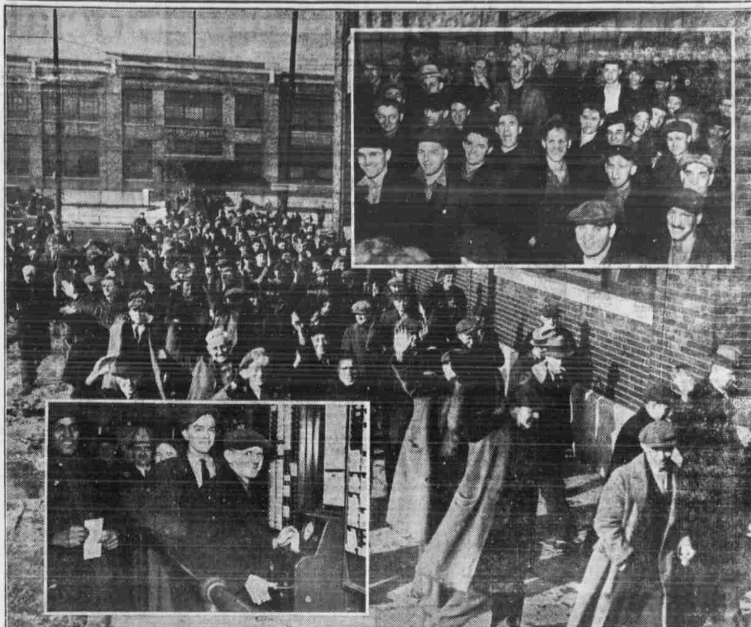
Approximately 90 per cent of the 40,000 Chevrolet workers called back to work last week reported at their work benches. Above is shown a group of happy Chevrolet workers as they return to their jobs at the Chevrolet Gear and Axle plant in Detroit, in line with the company's program of giving part-time employment to as many employees as possible in order to keep
