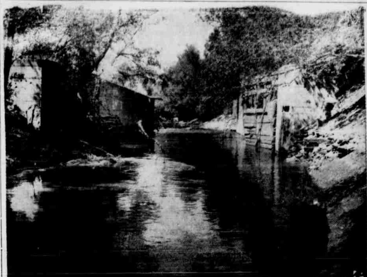
DALLAS' STEAMBOAT LOCKS The locks are on the Dr. James J. Hamiter place a mile down the Trinity River from the Dallas city limits. The concrete is about four years old when Dallas had dreams of being a riverboat town. The gates are loose on their hinges. The locks are now submerged when the river is a flood. —AP Photo
