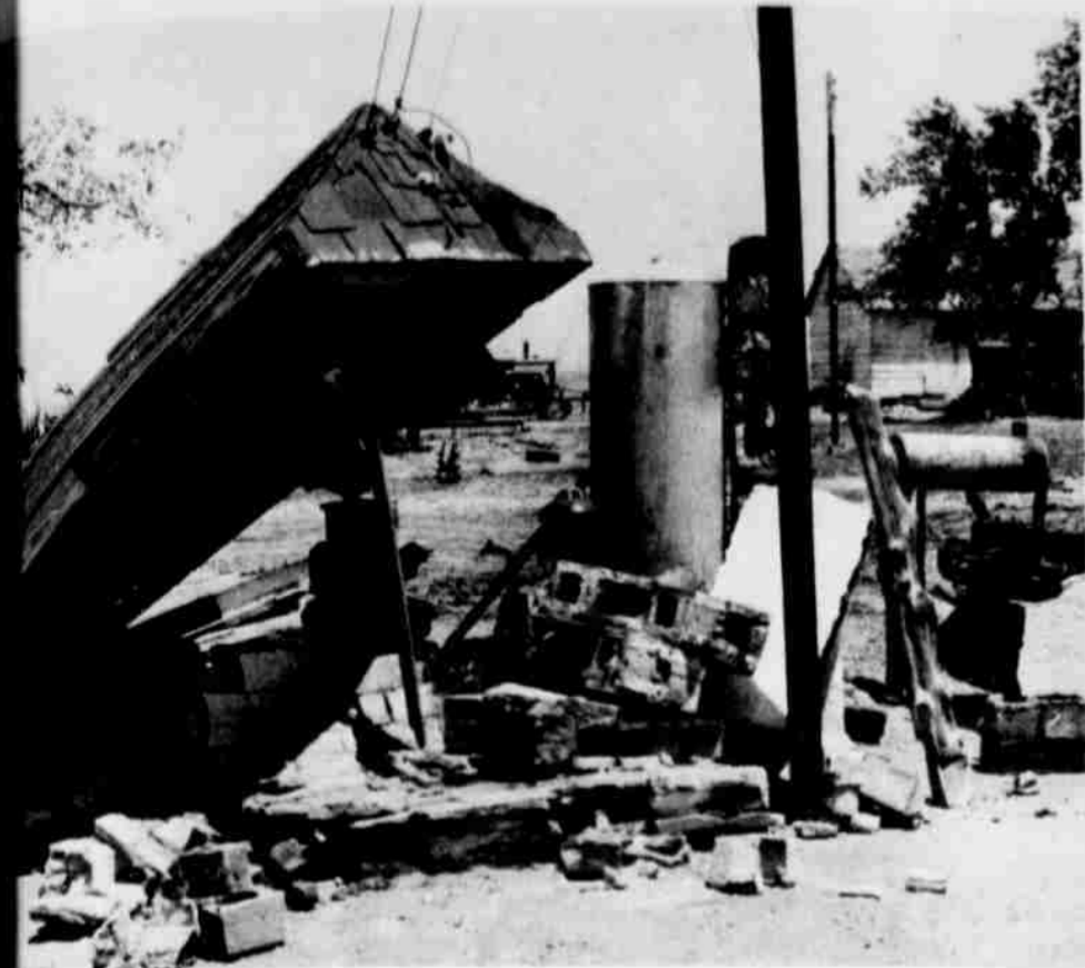
HOUSE DESTROYED — Pictured above is what remains of a well house on the Geanphenson farm north of Whitharral after a small tornado struck Thursday afternoon. Other also damaged buildings at the O. L. Martin farm west of Stephenson's.
