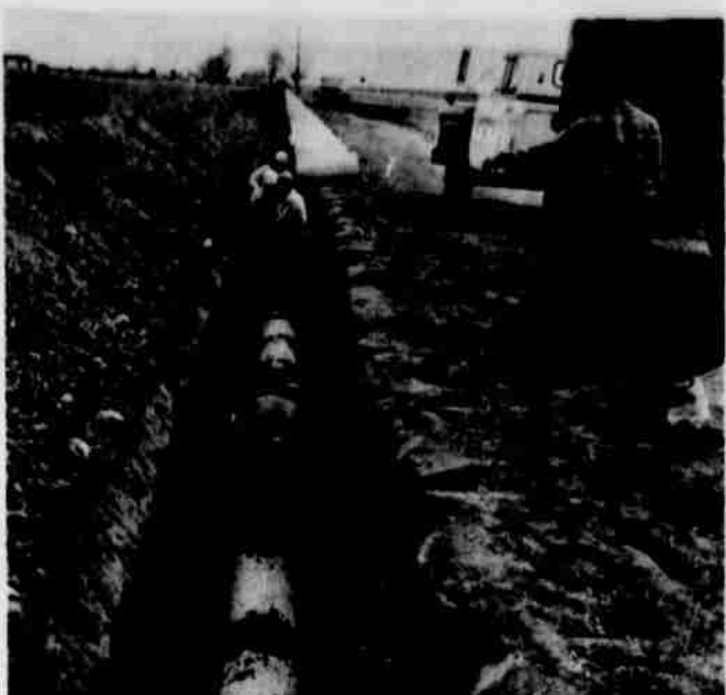
DOWN GOES THE LINE--Installation of a 12-inch underground concrete irrigation pipe is shown underway at the D.J. Hoose farm, four miles north of Springlake.
